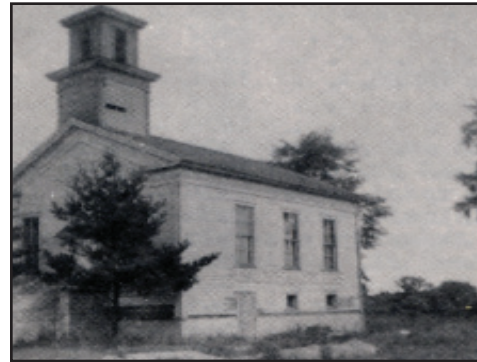
3 Raised again for a new foundation in 1951.
