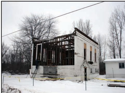
9 Roof trusses and front siding removed 1/14/2011.
