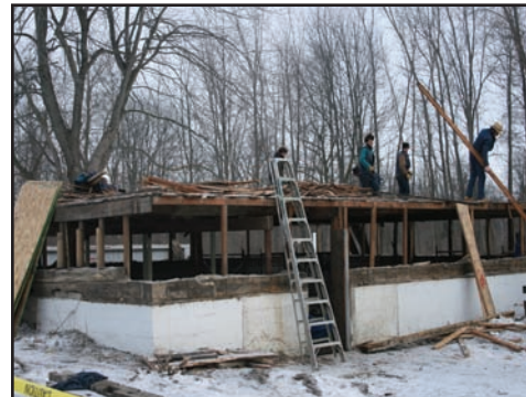
11 Upper walls removed 1/20/2011.
