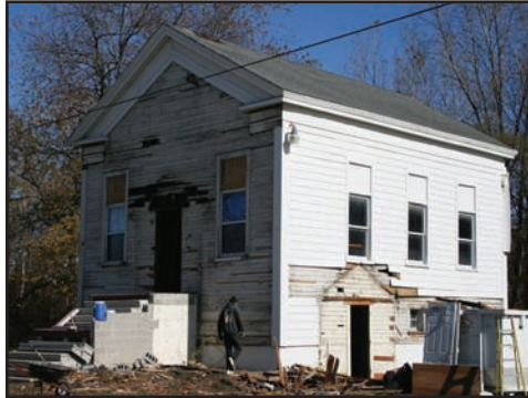
6 Covered porches removed 10/19/2010.
