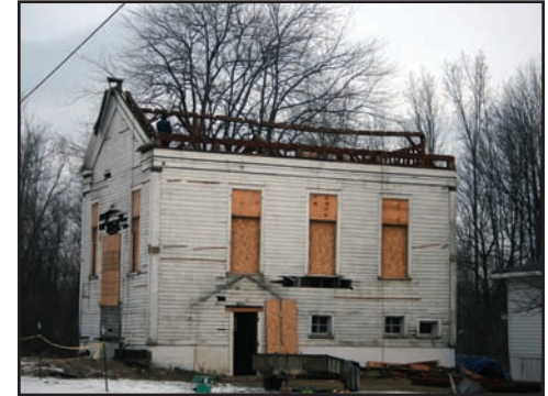
8 Contractor begins dismantling 1/10/2011.
