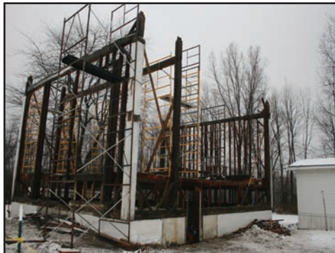
10 Side walls and cross beams removed 1/18/2011.
