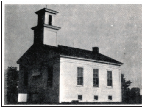
2 Church after the floor was raised in 1930.
